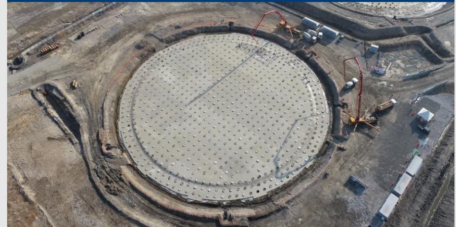
TK-202 Bottom Concrete Reinforcement
