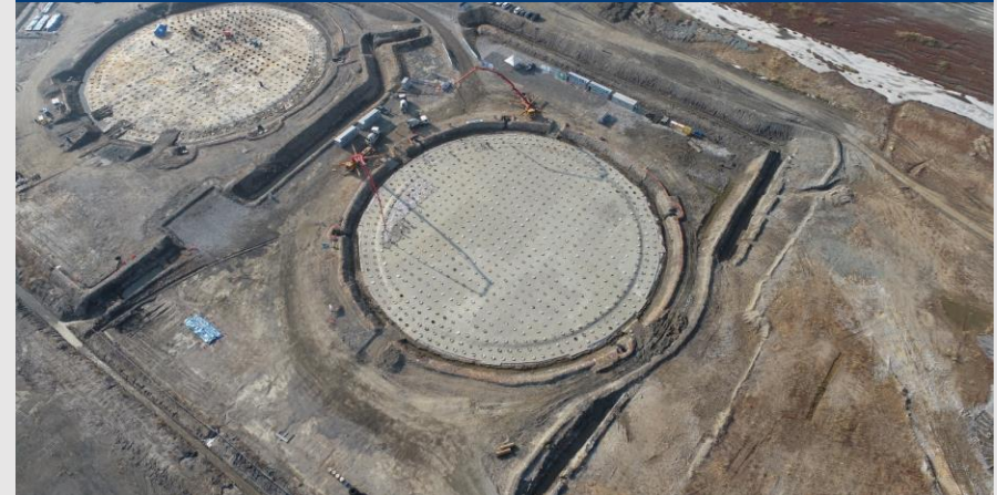
TK-202 Bottom Concrete Reinforcement
